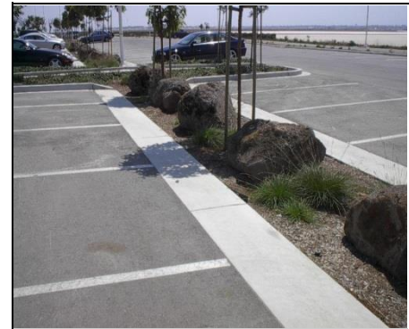
Infiltration islands in parking lots can help reduce stormwater runoff.
